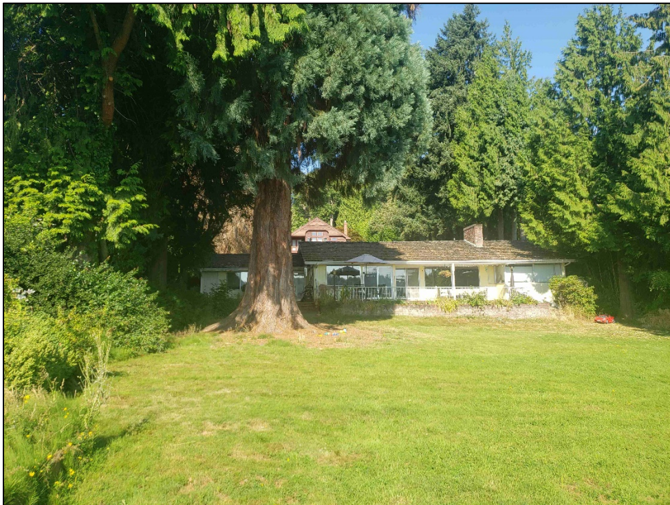
Figure 1. Subject property, existing residence, facing west
